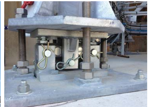
Load cells for skirted silo
