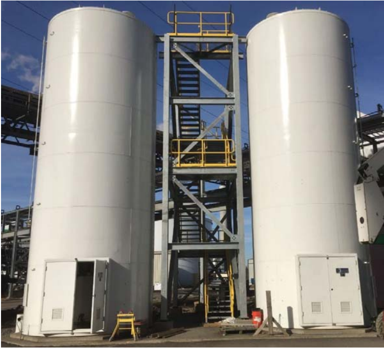
Redundancy with stairway to access on both roofs
